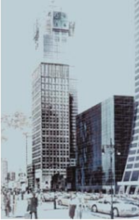
4 Times Square in New York City is one of the first office buildings in the U.S. to be powered by a 200 kW phosphoric acid fuel cell system (Courtesy: International Fuel Cells)
